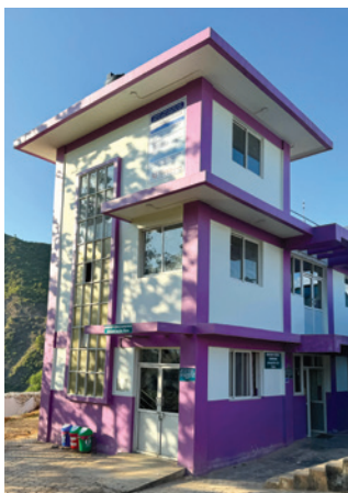
Emergency entrance at Chaurjahari Hospital in Chaurjahari, Rukum, Nepal
